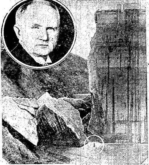
The shattered remains of the giant St. Francis Dam, near Newhall, Calif., released 12,000,000 gallons of water to flood the Santa Clara valley, is pictured above. Many huge chunks of concrete thousands of tons were carried three-quarters of a mile by the irresistible wall of water.
